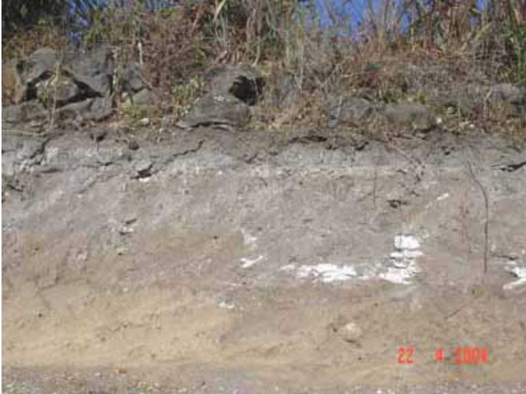
Figure 9. CZ-116. Profile showing a house foundation.
