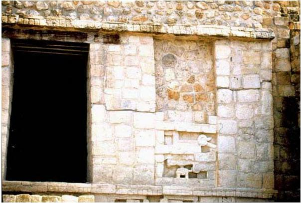
Photo 29. Ek Balam, Temple 1, detail of partially empty joints to divide the integrated parts from the original ones, August 1, 2000.
