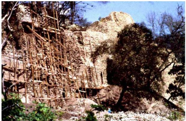
Photo 64. Copán, archaeological cut, in the process of stabilization. Wooden scaffolds were used throughout the entire work, 1992.
