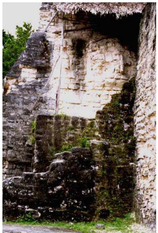
Photo 48. Tikal, Structure 5D-22, idem photo 47, though this one was taken on December 13, 2000; note that the mask has almost disappeared. The damp parts with a heavy dark color show a much better state of preservation than the roofed portion.
