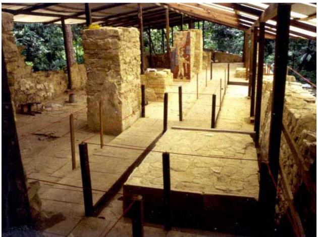
Photo 57. Palenque, Structure XIX after restoration was completed. There is a footpath for tourists and a protective roof. There are no side walls and therefore ventilation is constant, while the shade of trees helps to stabilize the interior temperature, July, 2000.
