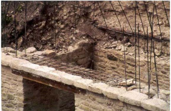
Photo 15. Cahal Pech, Structure 19 during reconstruction, using numerous iron bars, June 12, 1992.
