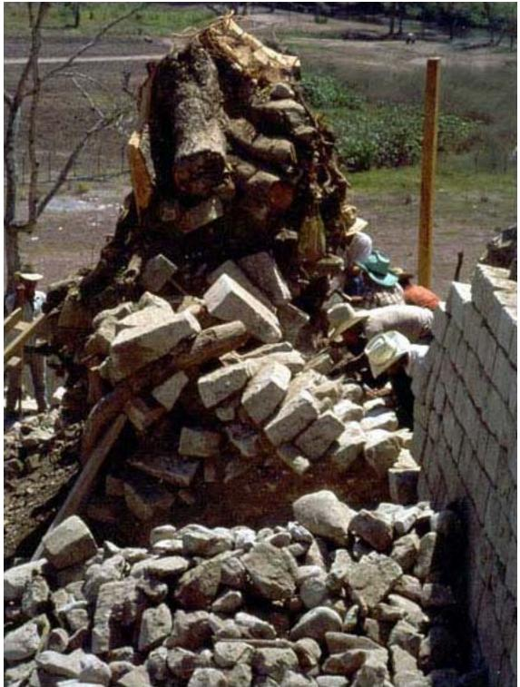
Photo 51. Copán, Structure 10L-21, north section, restoration process through anastylosis, March, 1991.
