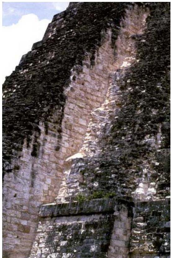
Photo 43. Tikal, Temple 1, south side of the stairs, heavily deteriorated; note the white dust on the joints with the terraces, May 14, 2000.
