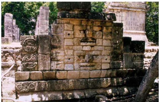
Photo 12. Chichén Itzá, NE colonnade. Repairs using anastylosis in adjacent space, July 31, 2000.
