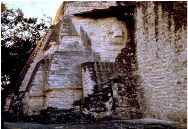
Photo 47. Tikal, Structure 5D-22, west mask. The light parts represent deterioration. The parts darkened by microflora are better preserved, February, 1978.
