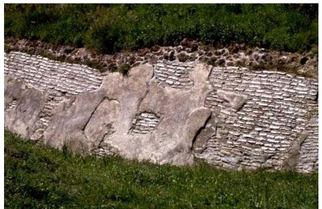
Photo 26. Cholula, restoration with the use of small stones in the joints to show the reintegrated portions, July 16, 2000.
