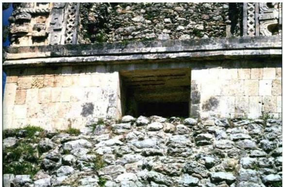
Photo 13. Uxmal, Quadrangle of Nuns. Deteriorated concrete lintel, July 28, 2000.
